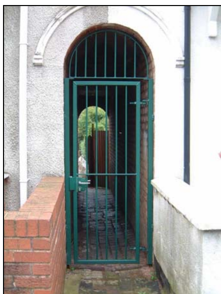
Figure 3.1: A lockable alley-gate installed as part of the Phase 1 - 19 SDP
